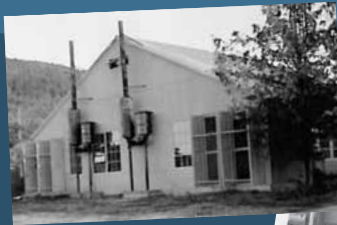
The first generating plant was completed for a total cost of $150,000
