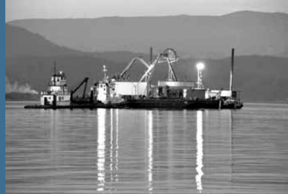
1993 Cable Lay Project, Steve Horn Photography
